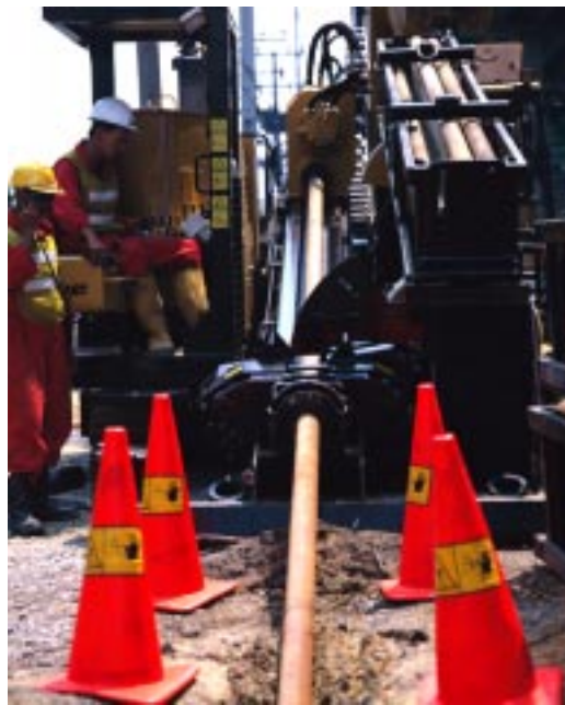
Drill rig crew confirming steering commands during off-track locating.
