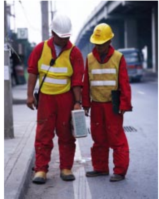
Locating on access road below on-ramp to Rangsit Pathumthani Highway.
