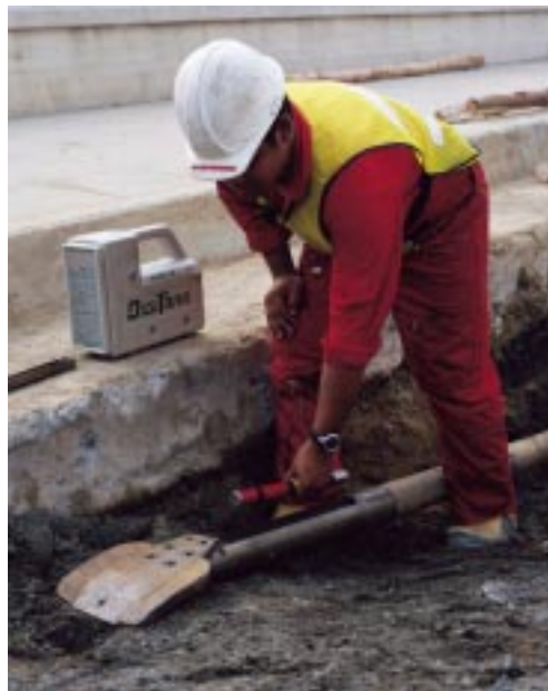
Transmitter being inserted into housing with extra-wide steering blade.
